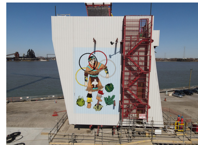
A mural depicting an Indigenous hoop dancer at the Canadian bridge site
