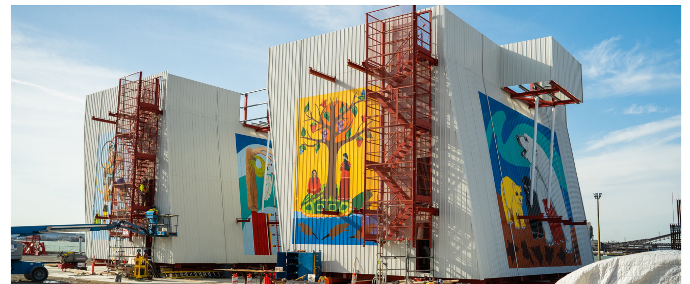
Art murals designed by Walpole Island First Nation and Caldwell First Nation artists installed at the Canadian bridge site
